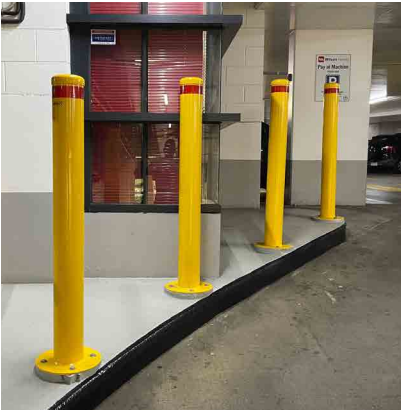
Surface Mount Bollards Installed for Wilson Security
