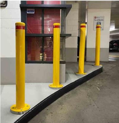
Surface Mount Bollards Installed for Wilson Security
