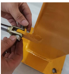
Step 5: Gas strut installation
