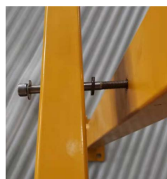
Step 3: Put arm connector through arm and post as per drawing above
